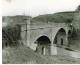
B2841 Fyansford Bridge
