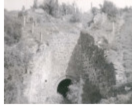
B1637 Lime Kiln Limeburners Point Geelong
