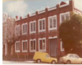
B5054 Classroom Block
