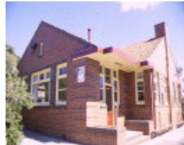
malvern primary school no 2586 tooronga road malvern domestic arts building
