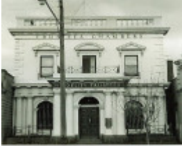
B0254 Former Colonial Bank Geelong
