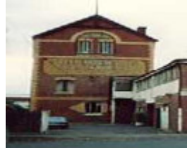
B5717 Friedrich & Bassemir Buildings
