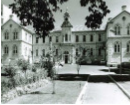
B1046 Old Base Hospital
