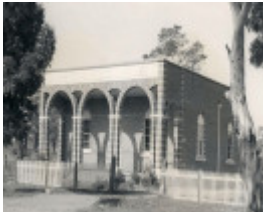
B1856 Old Shire Council Chambers
