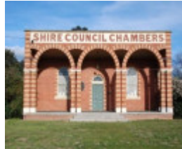
B1856 Old Shire Council Chambers
