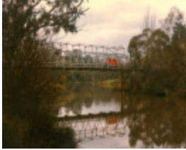
B6852 Queens Park Bridge North Side
