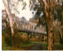
B6852 Queens Park Bridge Geelong
