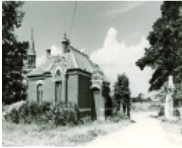
B5048 Gatehouse St Albans Homestead
