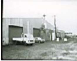
B5727 Central Foundry Pty Ltd
