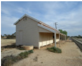
MANANGATANG RAILWAY STATION COMPLEX SOHE 2008
