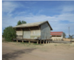
MANANGATANG RAILWAY STATION COMPLEX SOHE 2008
