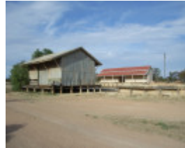
MANANGATANG RAILWAY STATION COMPLEX SOHE 2008
