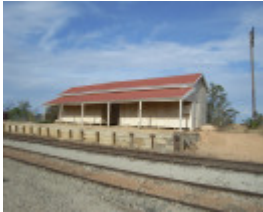
MANANGATANG RAILWAY STATION COMPLEX SOHE 2008
