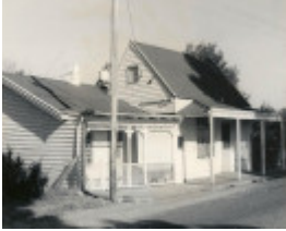
B1267 Former Post Office 197 Main Rd Hepburn Springs
