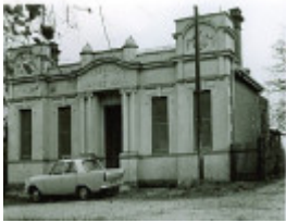
B5844 Former Creswick Shire Hall
