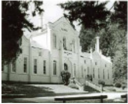
B0022 Frmr Hospital, Frmr School of Forestry
