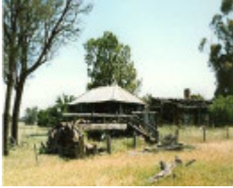
B5774 Homestead Outbuildings & Cool Room
