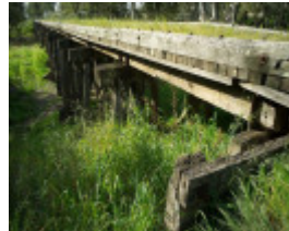
B6910 Wimmera River Rail Bridge
