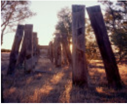
B6910 Wimmera River fmr 12 span bridge
