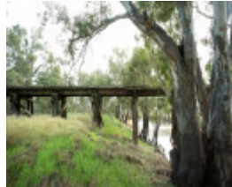
B6910 Wimmera River Rail Bridge
