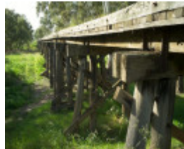
B6910 Wimmera River Rail Bridge
