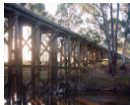
B6910 Wimmera River Rail Bridge
