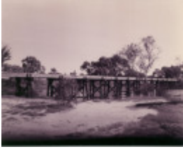
B6910 Wimmera River Rail Bridge
