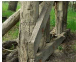
B6910 Wimmera River Rail Bridge
