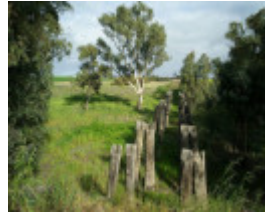
B6910 Wimmera River former 12 span bridge
