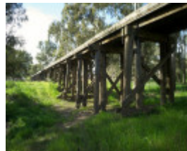
B6910 Wimmera River Rail Bridge
