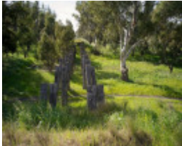
B6910 Wimmera River former 12 span bridge
