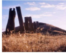
B6910 Wimmera River fmr 12 span bridge
