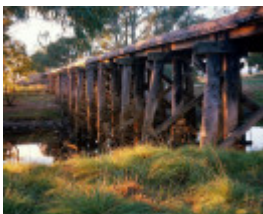
B6910 Wimmera River Rail Bridge
