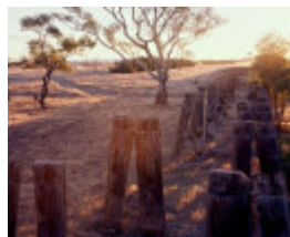
B6910 Wimmera River fmr 12 span bridge
