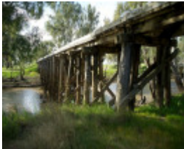
B6910 Wimmera River Rail Bridge
