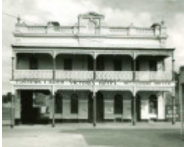
B2184 Cast Iron Verandahs
