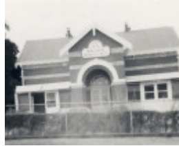
B0622 Ovens & Murray Hospital for the Aged Beechworth
