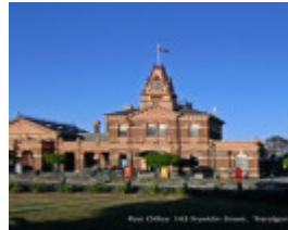
B2722 Court House & Post Office
