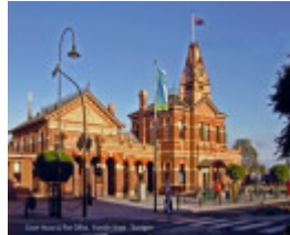
B2722 Court House & Post Office
