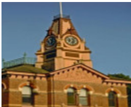
B2722 Court House & Post Office
