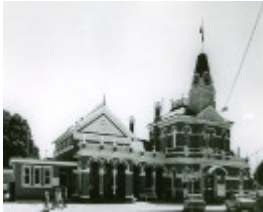
B2722 Court House & Post Office
