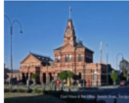
B2722 Court House & Post Office
