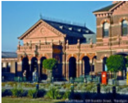
B2722 Court House & Post Office
