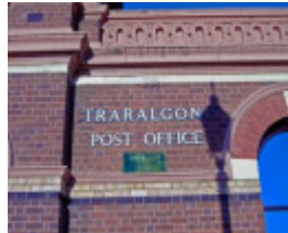
B2722 Court House & Post Office
