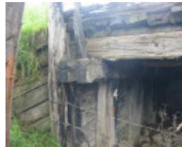
B6954 Tyers Road Bridge abutment
