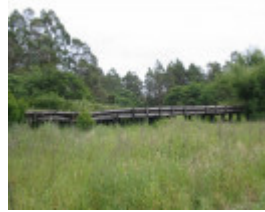
B6954 Tyers Road Bridge
