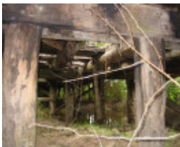
B6954 Tyers Road Bridge substructure
