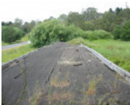
B6954 Tyers Road Bridge deck
