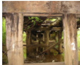
B6954 Tyers Road Bridge piers
