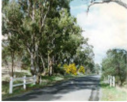
B6922 Masonry & Timber Culvert
