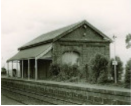
B5319 Goods Shed, Riddell's Creek station
