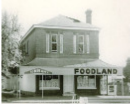
B3576 Former Corner Store
