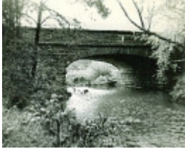
B0659 Woodend Bridge
