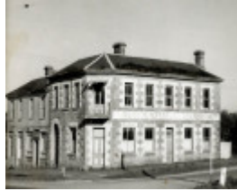
B1493 Former Hotel Malmsbury
