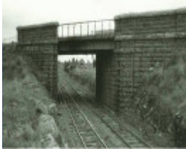
B7196 Bluestone Bridge
