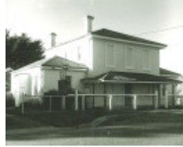
B2086 Former Court House & Police Station
