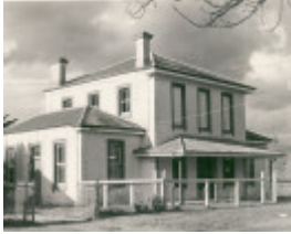
B2086 Former Court House & Police Station
