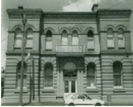
B0912 Former Colonial Bank
