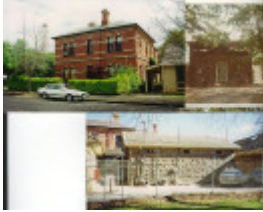
B6041 Former Police Station Gaol & Courthouse
