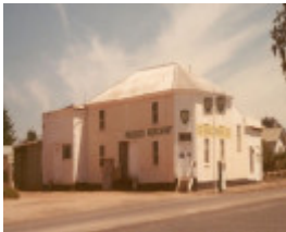
B4609 Wiegards Buildings (rear view)
