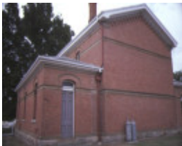
mansfield court house rear elevation feb1985
