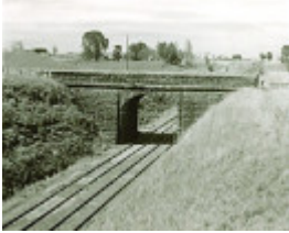
B4646 Road Bridge Malmsbury
