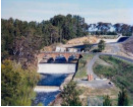
B6766 Upper Coliban Spillway Bridge
