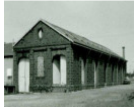
B3847 Kyneton Railway Station Goods Shed
