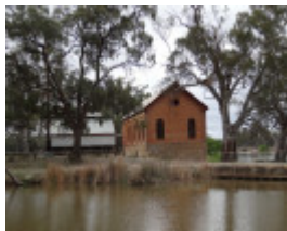
B3577 Psyche Bend pump house
