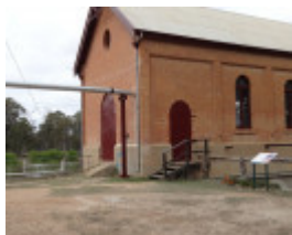
B3577 Psyche Bend pump house
