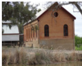
B3577 Psyche Bend pump house
