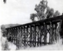
B3053 Railway Bridge
