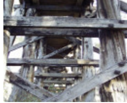
B3287 Railway Bridge Pyalong
