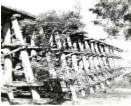
B3287 Railway Bridge Pyalong
