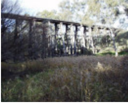
B3287 Railway Bridge Pyalong
