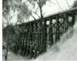
B3287 Railway Bridge Pyalong
