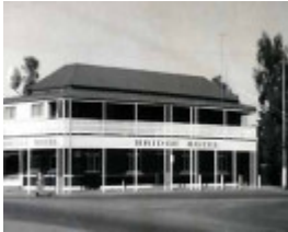
B2389 Bridge Hotel Nathalia
