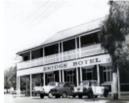
B2389 Bridge Hotel Nathalia
