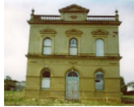
B4123 Former Mechanics' Institute
