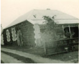
B4288 Former Bluestone Police Station
