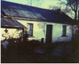
B5548 Ellerslie Cottage & Storeroom
