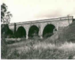
B2659 Railway Viaduct Barkers Creek
