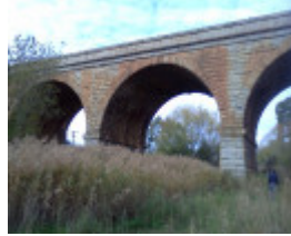
B2659 Railway Viaduct Harcourt 2012
