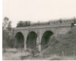
B2659 Railway Viaduct Harcourt
