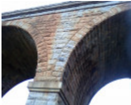
B2659 Railway Viaduct Harcourt 2012 detail
