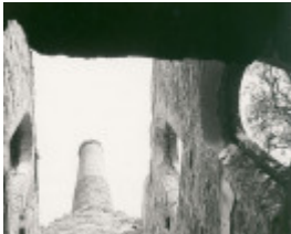
B1762 Ruins of Duke of Cornwall Mine
