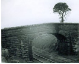
B2993 Humped Bridge Calder Hwy Taradale
