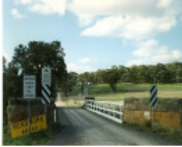
B6850 Zeal Bridge
