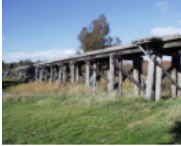
B6955 Winters Flat Bridge
