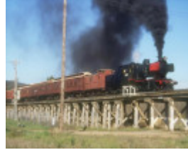
B6955 Winters Flat Bridge
