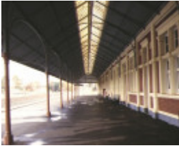
maryborough railway station platform view
