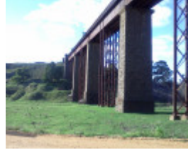
B1234 Taradale viaduct
