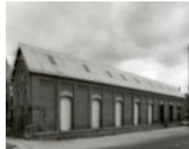
B3849 Goods Shed East View
